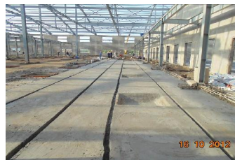
Construction of buffer concret and moisture release
