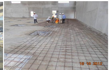
Insertion of steel on the warehouse floor
